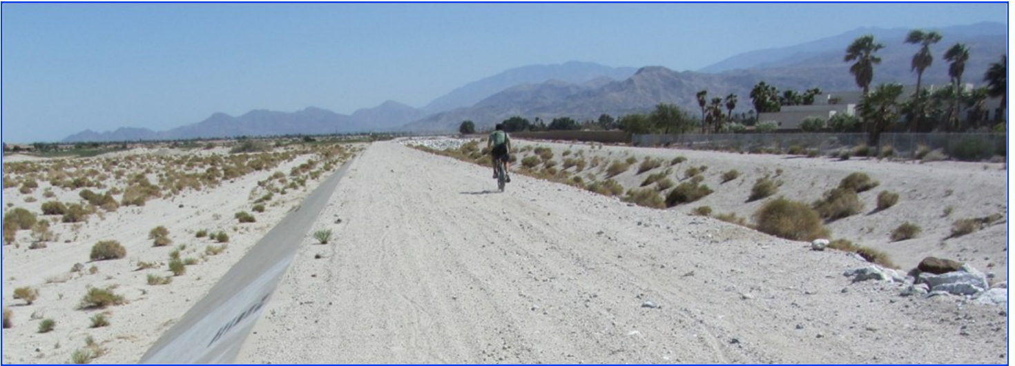
Figure 1. Existing levee along the Whitewater River (source: Alta Planning + Design).
